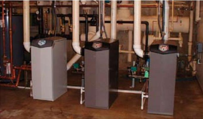
Designer Don Smet installed two Lochinvar Knight 500,000 BTU mod/con boilers and a Lochinvar Armor mod/con water heater with 399,000 BTU together in the main building. Photo courtesy of Lochinvar.
